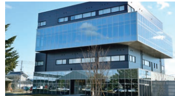
Training Facility Guest House
